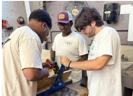
Several GENTs are finishing the cart box.
