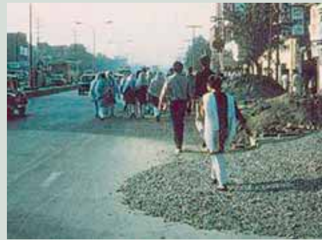
Figure 2.10 Pedestrians are forced to walk past a construction site in India because no facilities for pedestrians are provided by the contractor
